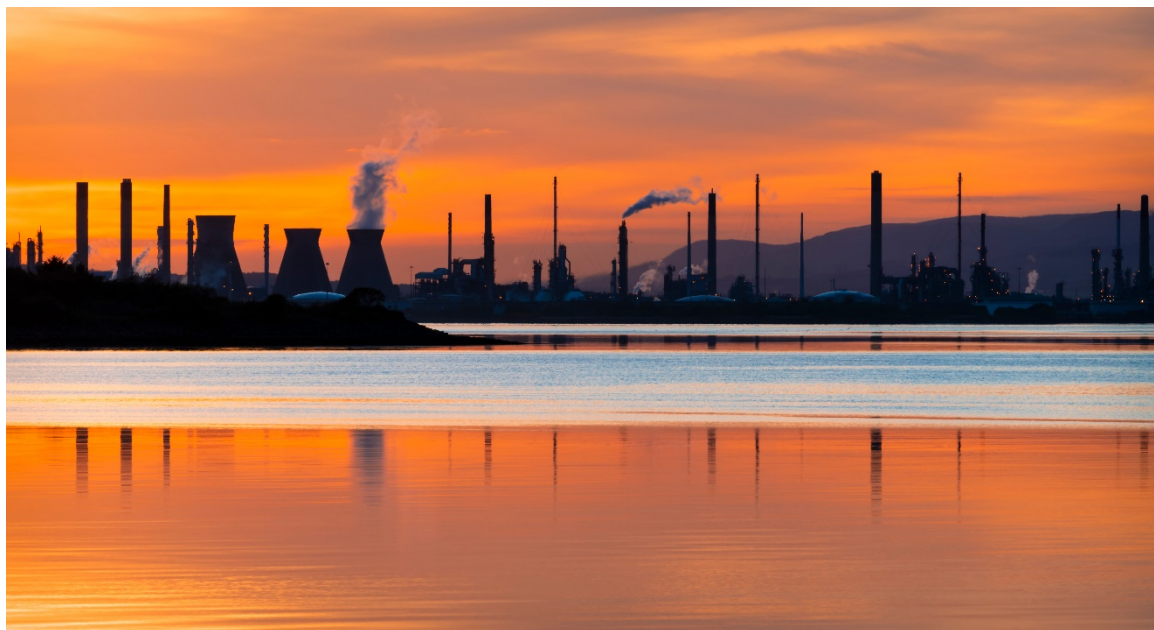
Ineos Grangemouth refinery
