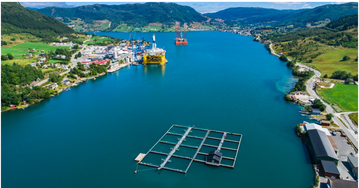
Oil and gas rig construction at Olen, Norway
